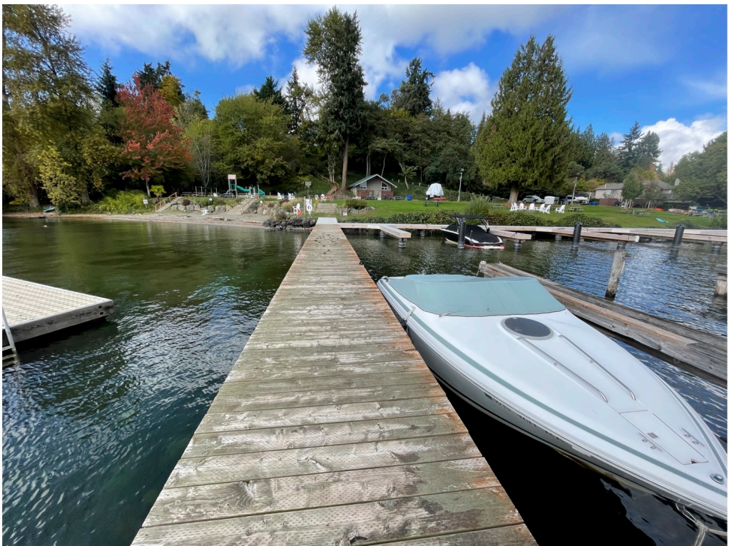
Photo 4 - Pier A looking landward.
