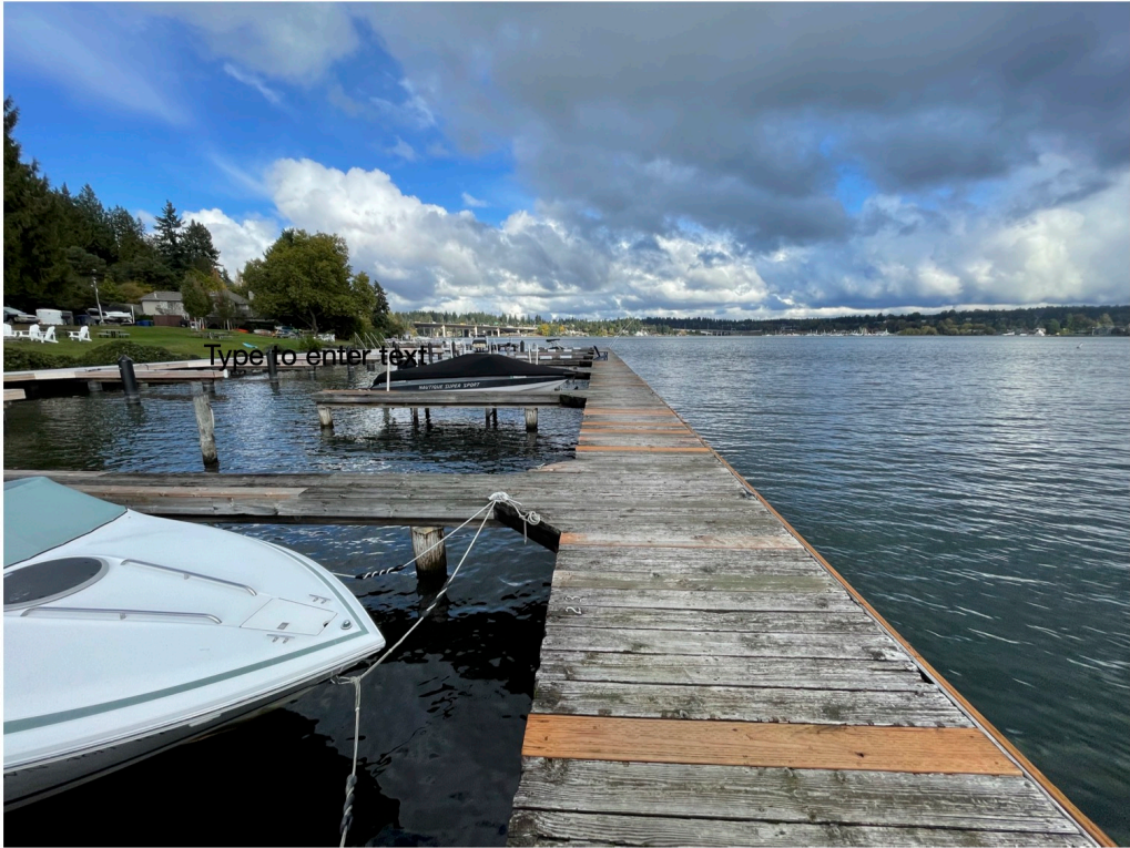
Photo 5 - Existing Pier A conditions.
