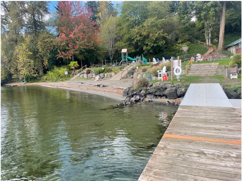
Photo 2 - Pier A looking landward showing shoreline conditions.
