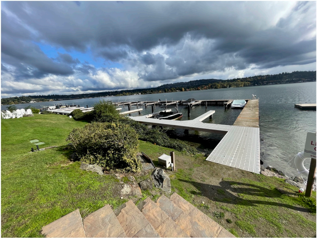
Photo 1 - Existing Pier A looking waterward.
