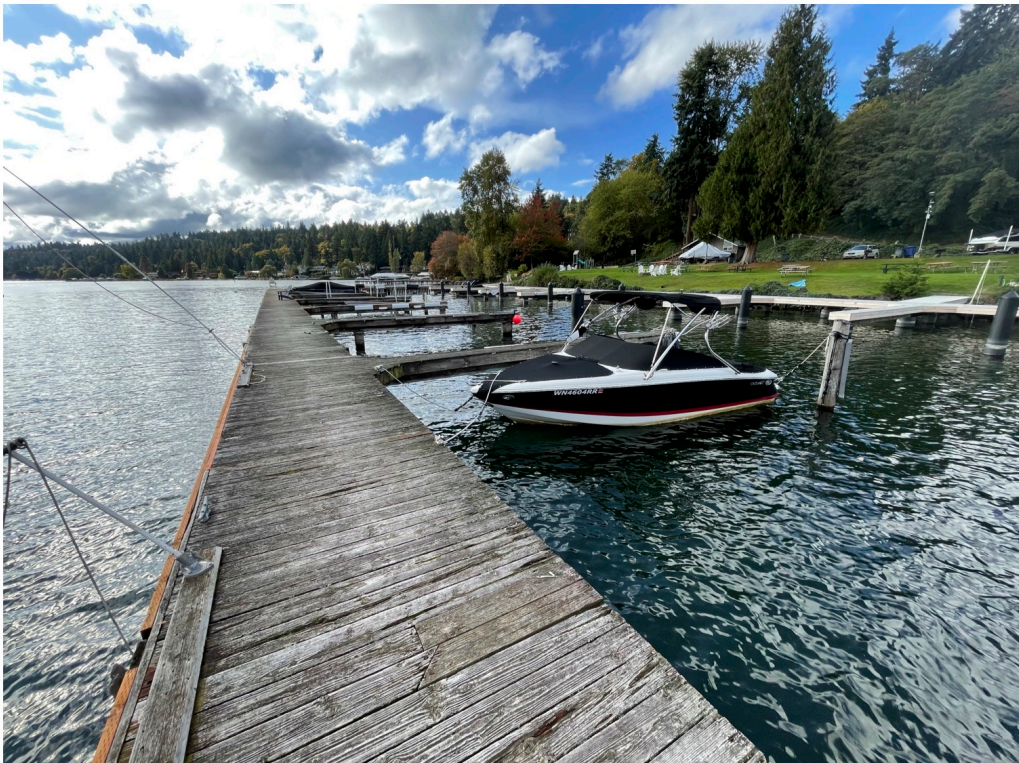
Photo 6 - Pier A existing conditions.
