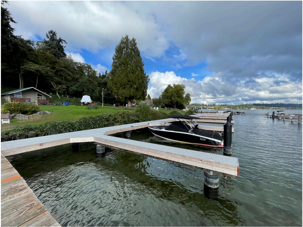
Photo 3 - Shoreline conditions along Pier A.
